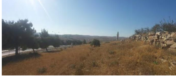
Figure A-5 Existing view from Viewpoint 5 (180° field of view): At-Tafilah is located on north of AEC wind farm.
